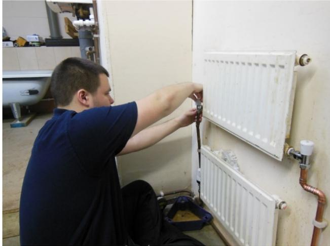
After isolating the heating system and draining it down the students will replace the valve that was leaking. Upon completion they will reinstate the water supply, fill, and vent the system before ensuring that the system is fully operational.
