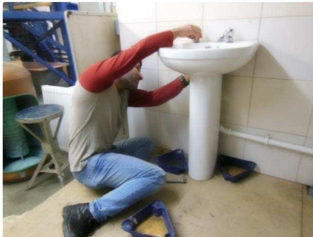
Replacing a defective basin pillar tap, this involves isolating the water supply and upon completion of work reinstating the water supply, testing for soundness (no leaks) and correct operation.
